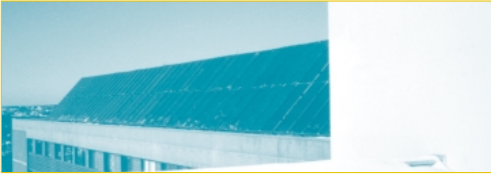
COLLECTORS ON TOP OF THE ROOF, MECANICAL ROOM LOCATED TO THE RIGHT.
