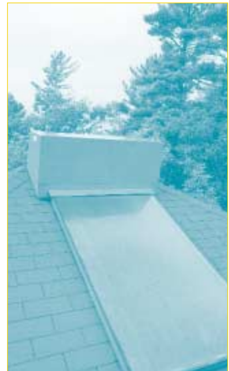
▲ Thermosiphon solar water heater at Camp Queen Elizabeth, Beausoleil Island on Georgian Bay, Ontario. Courtesy of Solcan Ltd.
